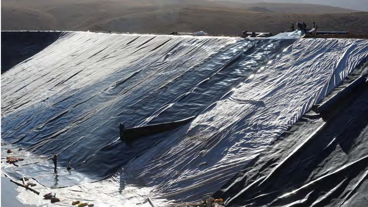
**Figure 2: Installing the liner on the 60,000m<sup>3</sup> water retention basin**
