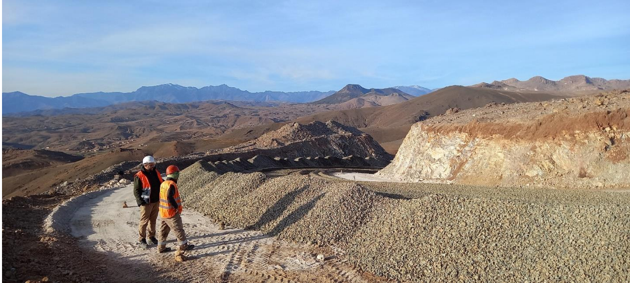
Figure 5 – Widening of the existing haulage road at Zgounder.
