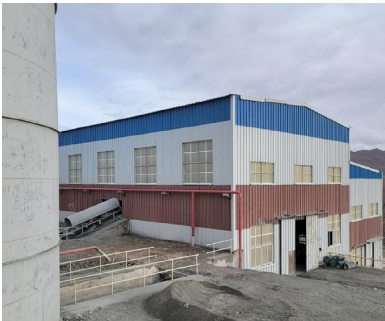
Figure 2: Installation of firefighting system at existing flotation plant
