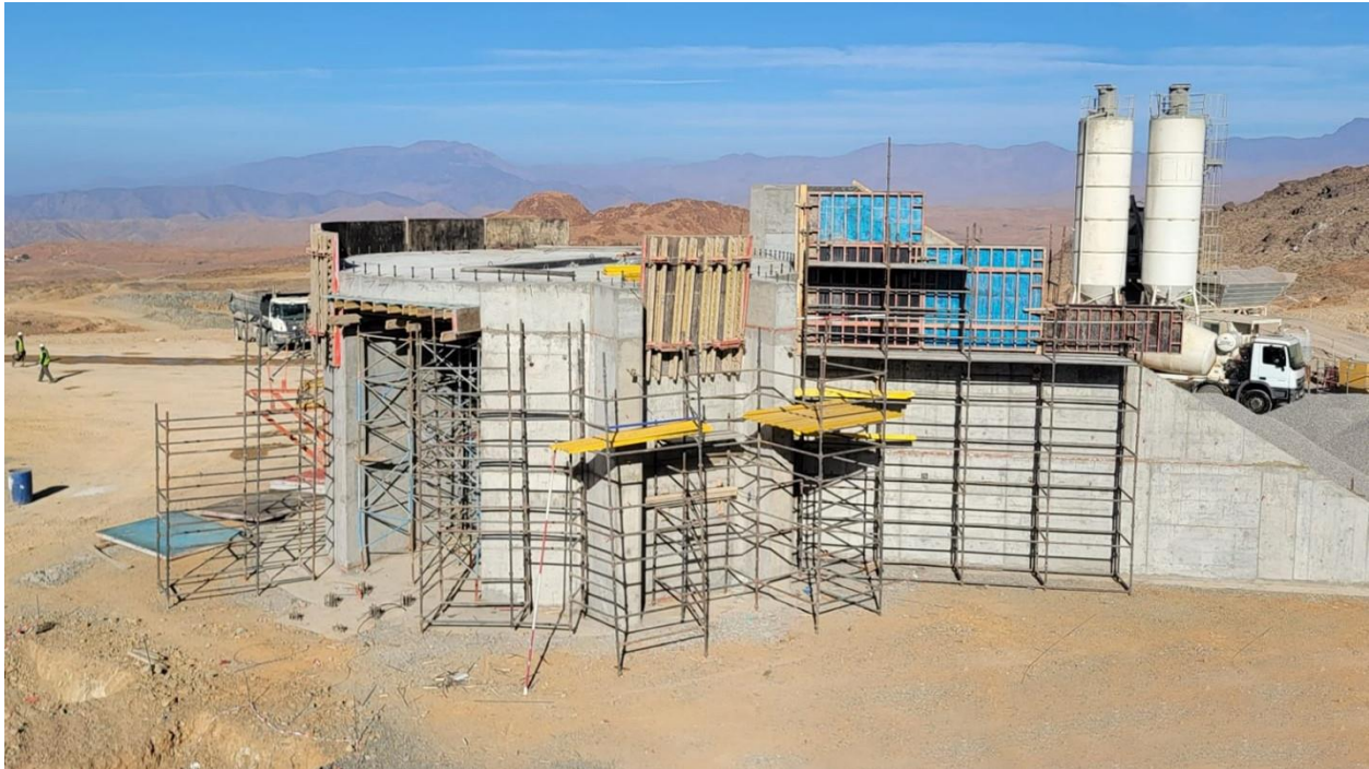
Figure 4: Ongoing construction of the ore silo
