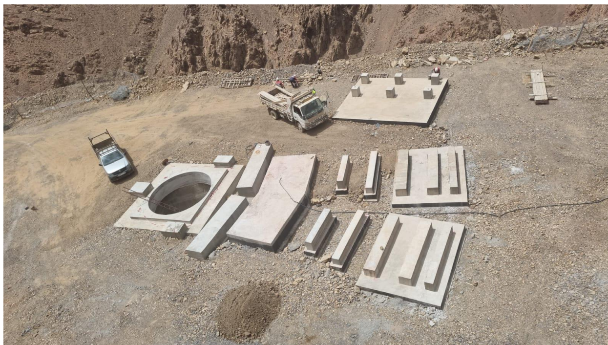
Figure 3: Completion of civil work for the ventilation shaft and equipment
