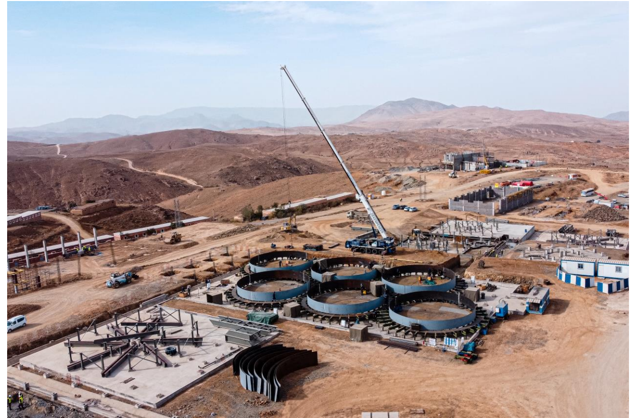
Erection of leach tank steelwork began in Q3
