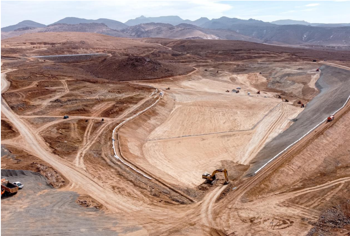
Tailings storage facility is near-complete
