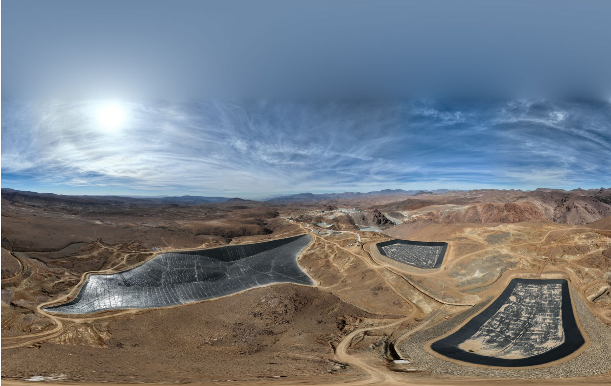
Tailings and water storage facilities are complete
