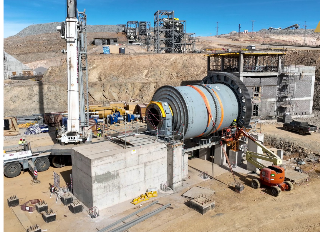
Installation of ball mill progressing well
