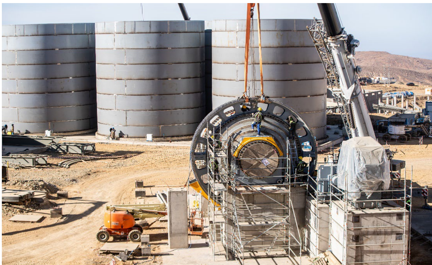
Figure 3: Ongoing Installation of the Ball Mill
