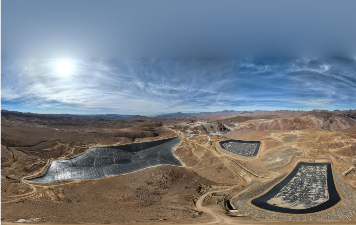
Tailings and water storage facilities are complete
