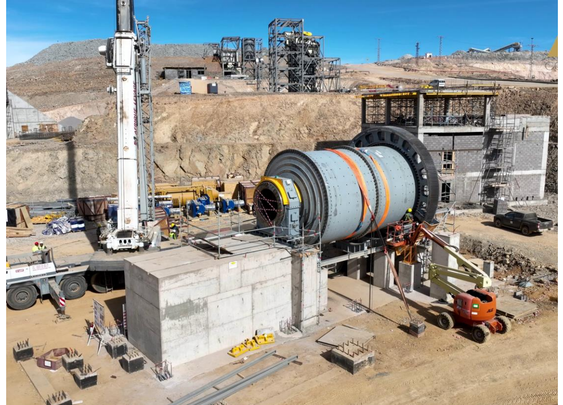
Installation of ball mill progressing well
